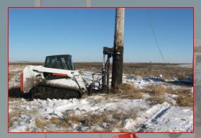
The Pole Jack removes all types of poles including foamed and cleated poles.
